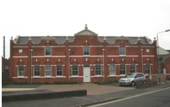
Figure 29: Early 20th century ironworks, New Borough Road.
