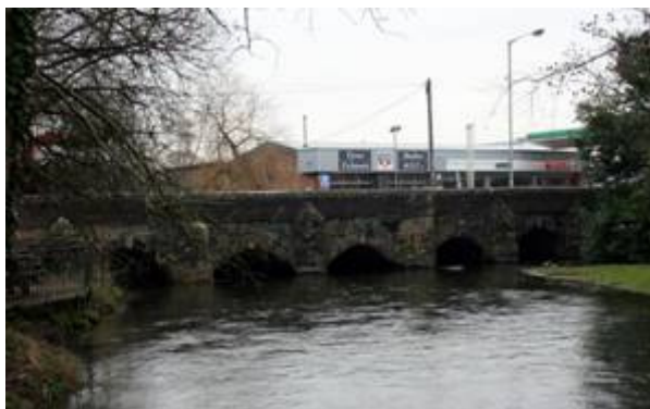
Figure 50: Walford Bridge, built in the early 16 th century
