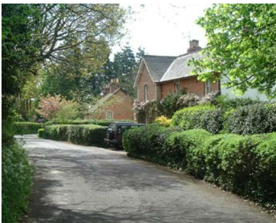
Victoria House, Sleight Lane
